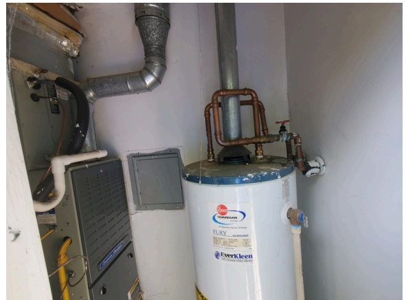
Fan-coil unit and water heater
