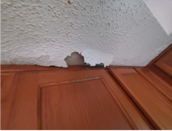
Typical ceiling peeling paint
